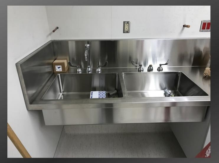
The installed sink fits neatly into to allotted location and plumbed for operation.
